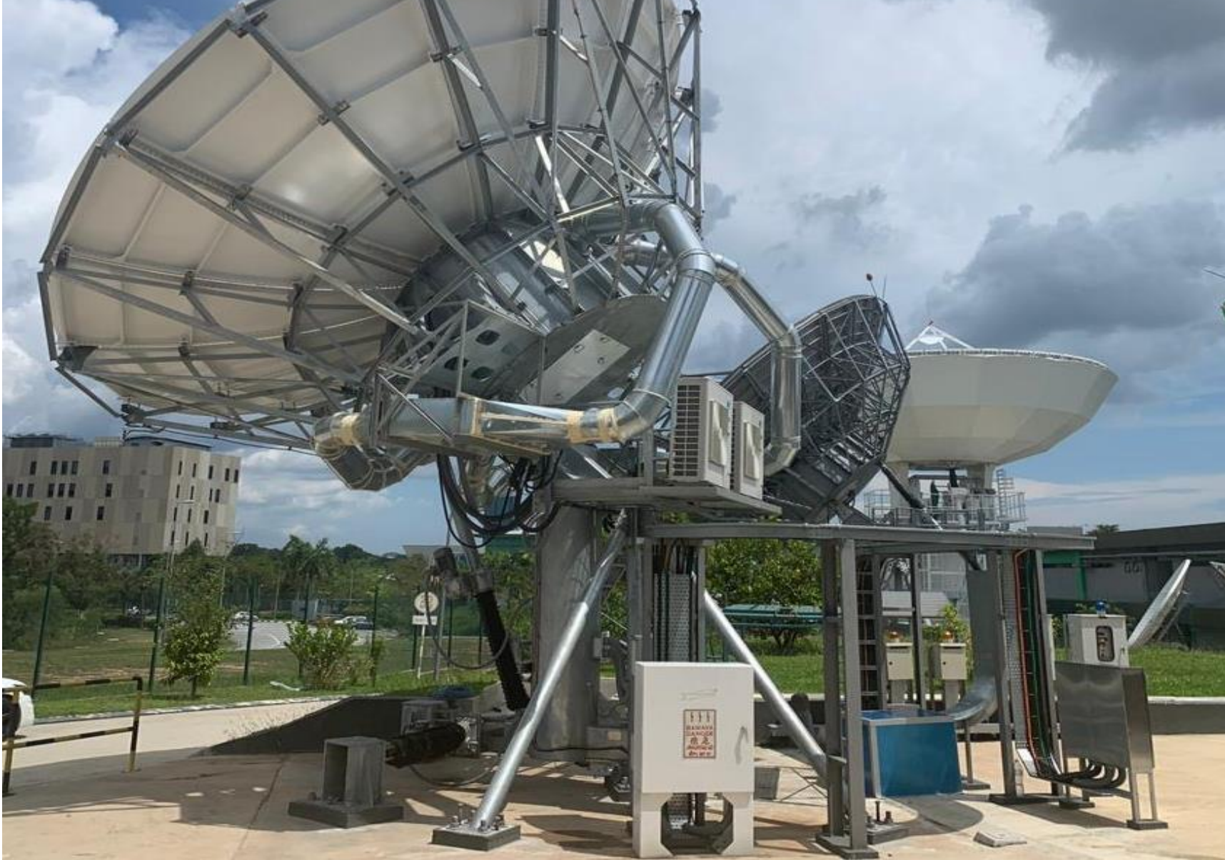
Unit 1: 7.3-mtr Ka-band Antenna TSGN Malaysia
