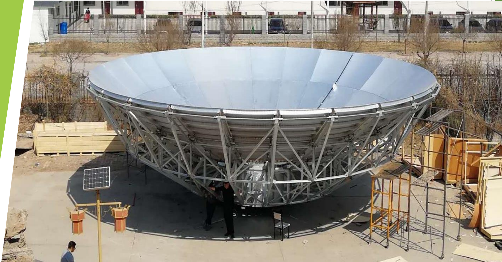
Initial Reflector Assembly
